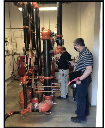
Overseeing annual fire pump inspections
