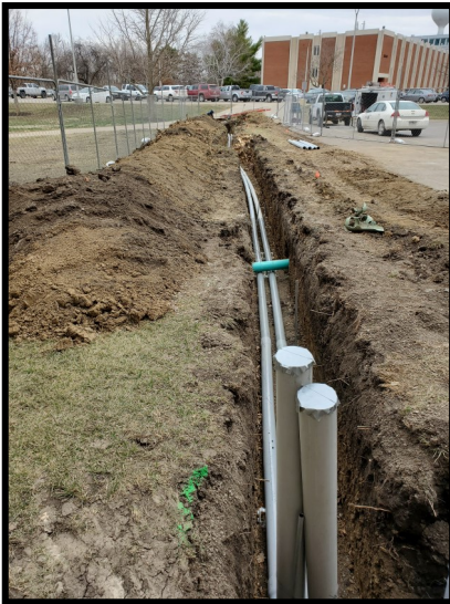
New power feed for Admin
