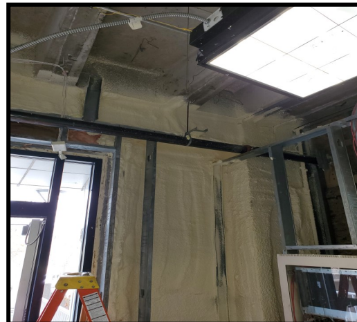
Garrett Strong fire main break repairs
