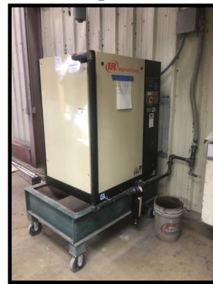
New Central Plant air compressor
