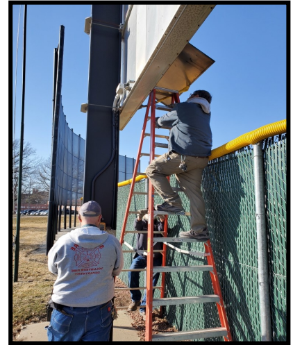
Electrical repairs to baseball scoreboard
